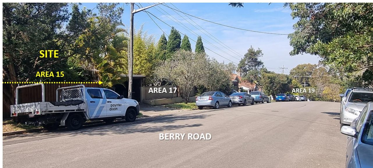
Figure 9: South of site at Areas 17 and 19. Facing south. (Source: Council Planner)
